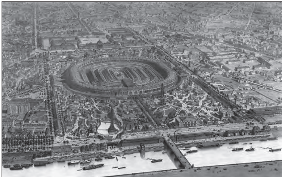
Fig. 8: Aerial drawing of the Champs de Mars of the 1867 Universal Exhibition in Paris (Source: Archives nationales, CP/F/12/11884/1).
